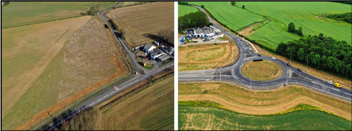
A46 Dunholme/Welton Roundabout – Before and After
