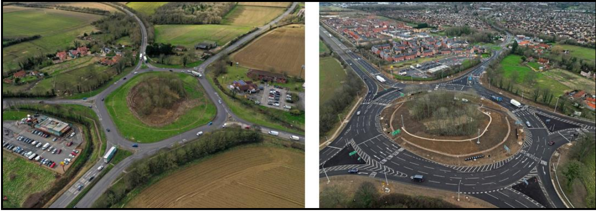
Holdingham Roundabout – Before and After
