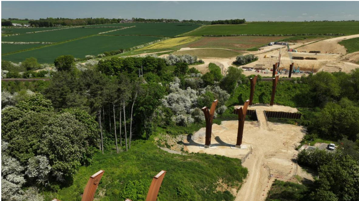
GSRR – Viaduct Piers Installed
